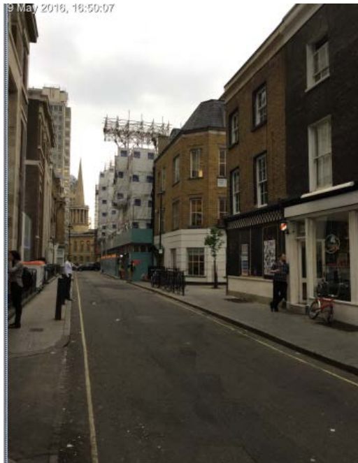
Street Context (North side of Riding House Street)
